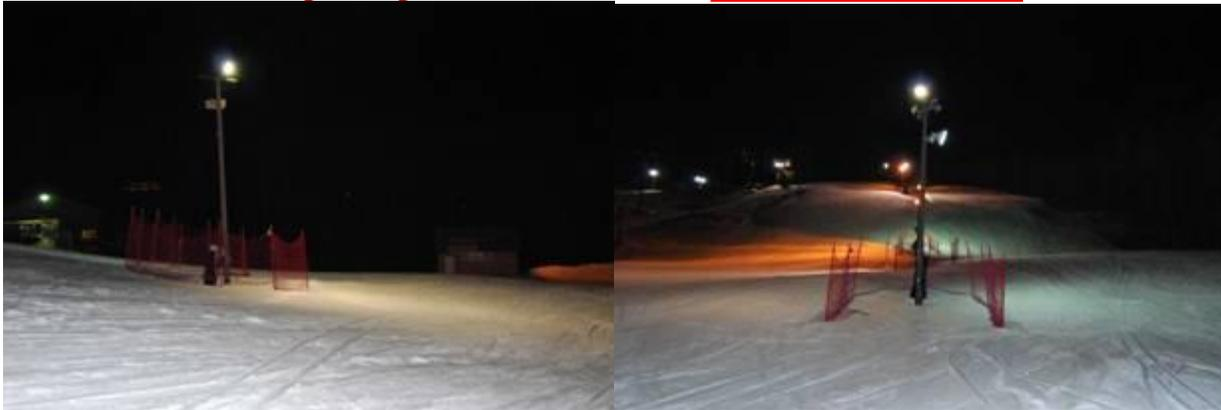
**The picture on the right demonstrates the difference between Snow-Bright and sodium. Notice the orange tint of the HPS fixture down the hill and to the left, compared the white light provided by the Snow-Bright™ fixture.**
