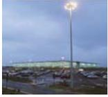
areas have been forced to use standard fixtures because that was all that was available. Some areas have resorted to high-mast configurations that are designed for roadways and fields. These lights can be mounted on poles ranging from 60-feet to more than 100-feet high. They produce an enormous
